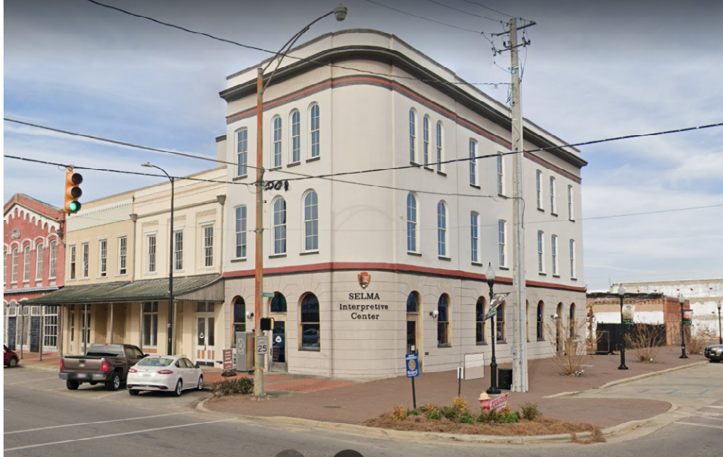
Street view showing 2 through 10 Broad Street (right to left) and the vacant lot with black privacy screen at 1119 Water Avenue (far right). Google, February 2022.
