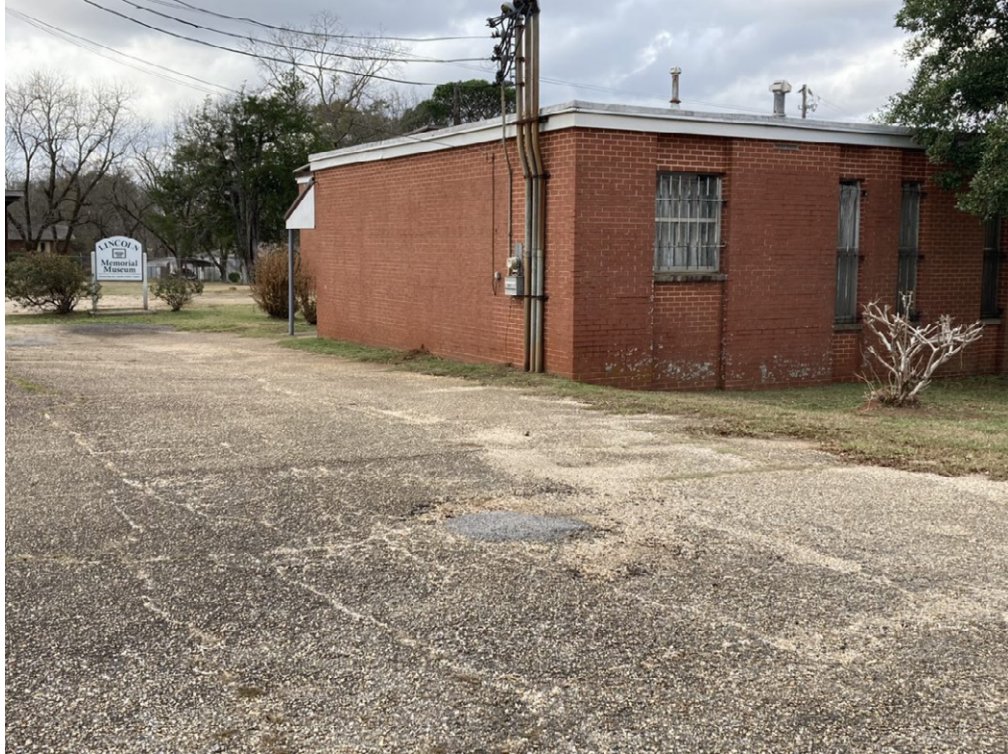
One-story classroom building with Lincoln Memorial Museum sign. NPS study team 2022.
