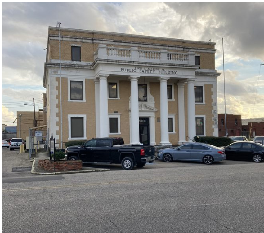
Cecil B. Jackson Public Safety Building. NPS study team 2022.
