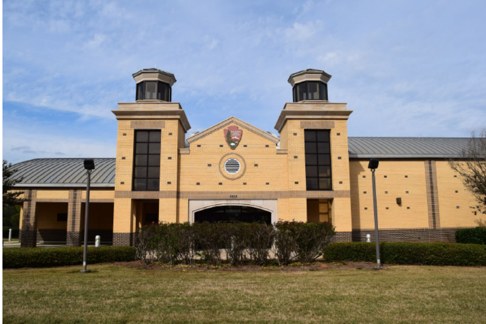
2020 photo of the south side of the Lowndes Interpretive Center. WLA Studio 2022. Figure 43.
