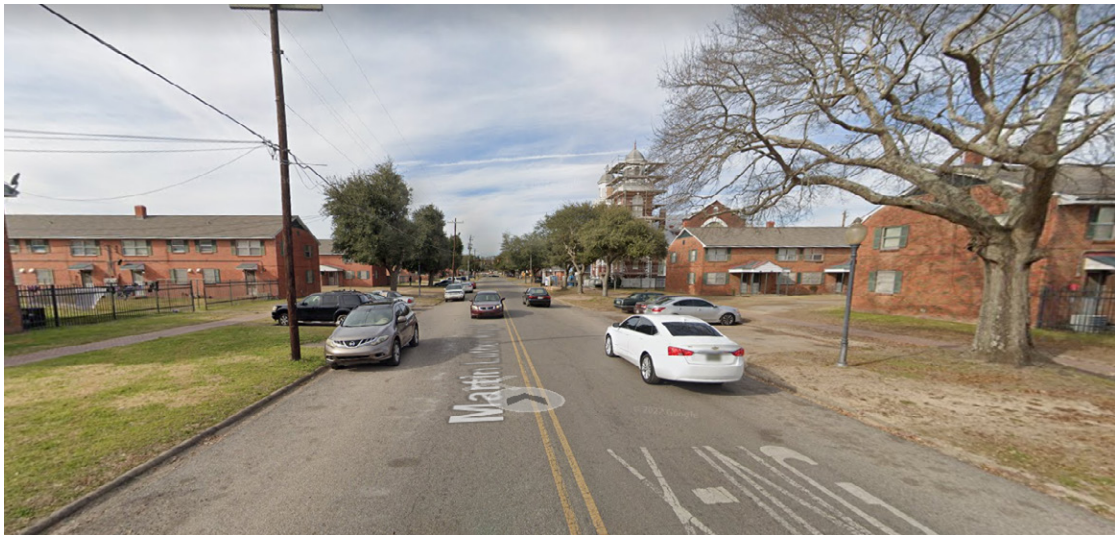
Street view of George Washington Carver Homes (left and right) with Brown Chapel A.M.E. Church in the background (with scaffolding) right of center. Google, February 2022.
