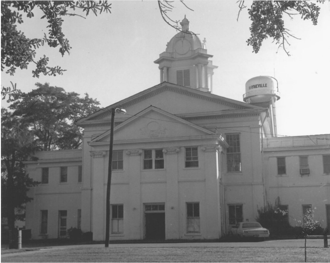
Front view of courthouse after alterations. W. Warner Floyd 1970. The photograph is part of the National Register nomination. Hand 1971.
