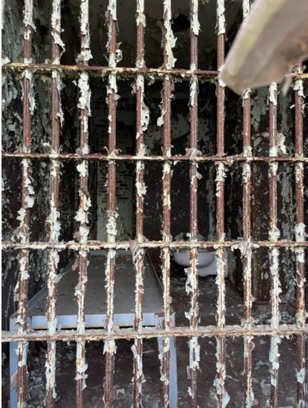
Interior of Old Perry County Jail. NPS study team 2022.
