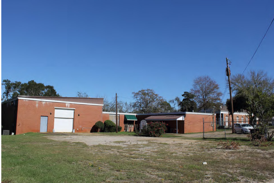
One-story classroom building. The photograph is part of the National Register nomination for the Lincoln Normal School. Causey 2020 in Pope Burns and Van West 2022.
