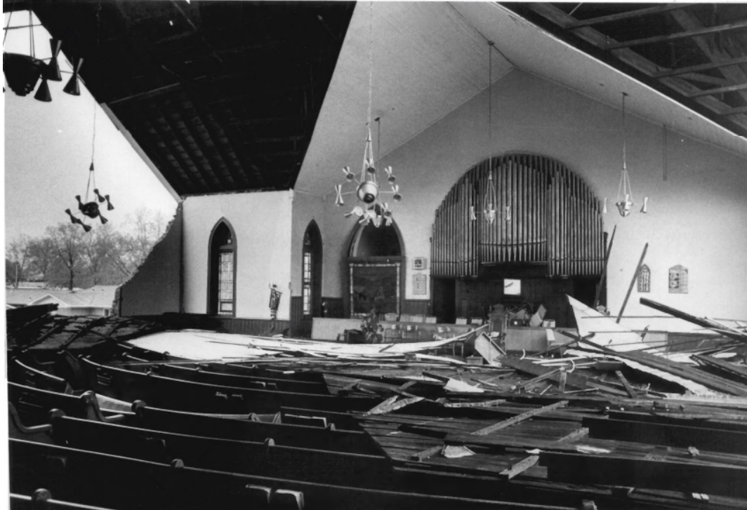
Interior, showing tornado damage. This photograph part of the National Register nomination for the First Baptist Church. Selma Times Journal (1978). Mertins 1979.
