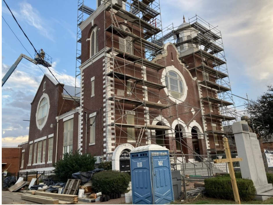
Brown Chapel A.M.E. Church under restoration. NPS study team 2022.
