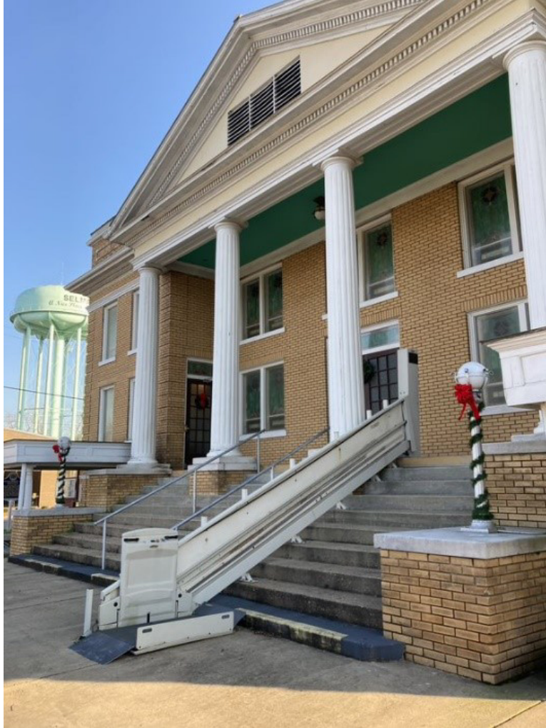
Tabernacle Baptist Church showing the Minter Avenue entrance and added chair lift. NPS study team 2022.
