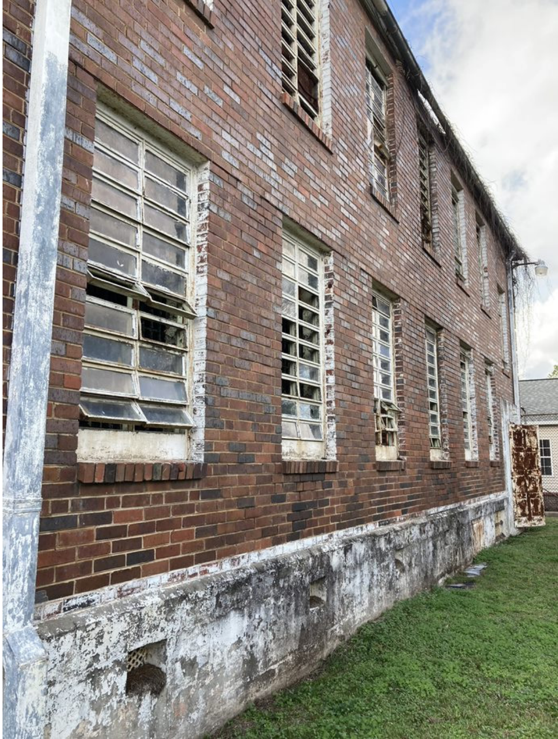
Old Perry County Jail rear of building. Window on left side of photo is visible from the jail cell where Reverend James Orange was held. NPS study team 2022.
