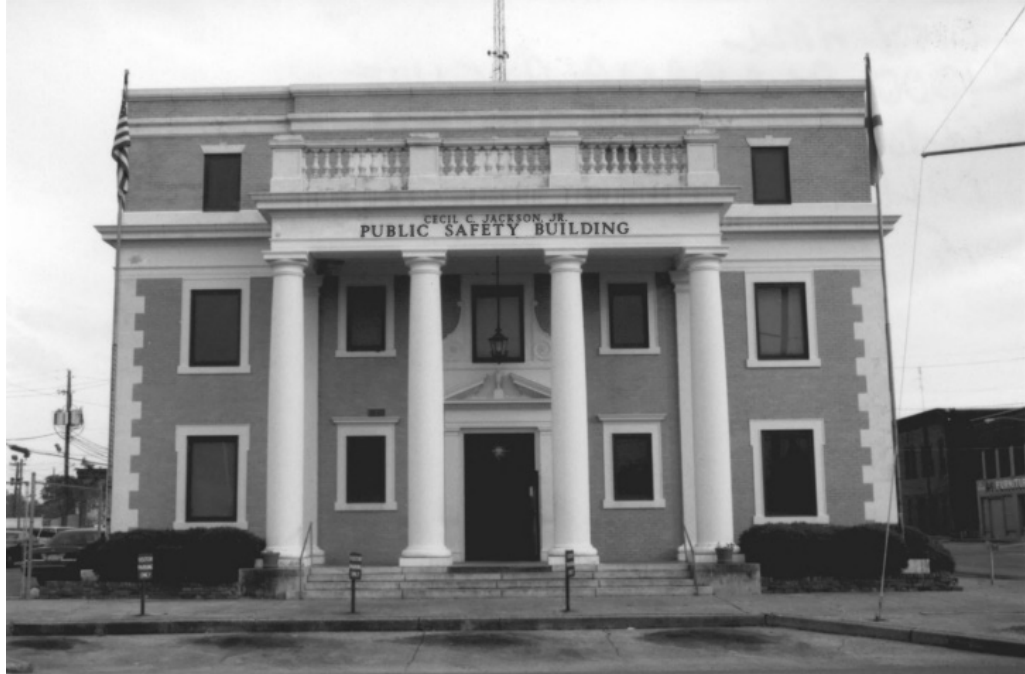
Cecil B. Jackson Public Safety Building. The photograph, taken in 2002, is part of the National Register nomination for the Old Town Historic District. Besser 2001.
