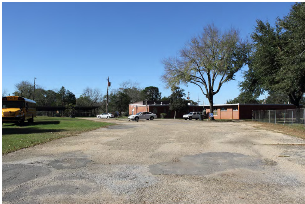
One-story classroom building. The photograph is part of the National Register nomination for the Lincoln Normal School. Causey 2020 in Pope Burns and Van West 2022.
