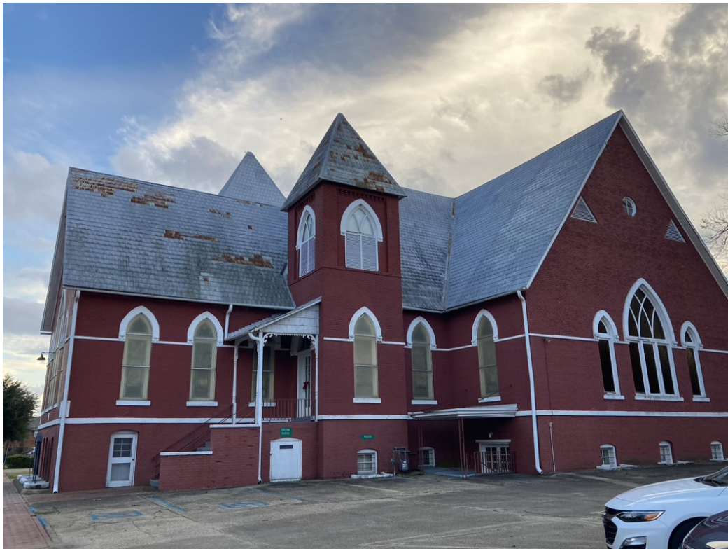
Exterior of First Baptist Church from the southwest. NPS study team 2022.
